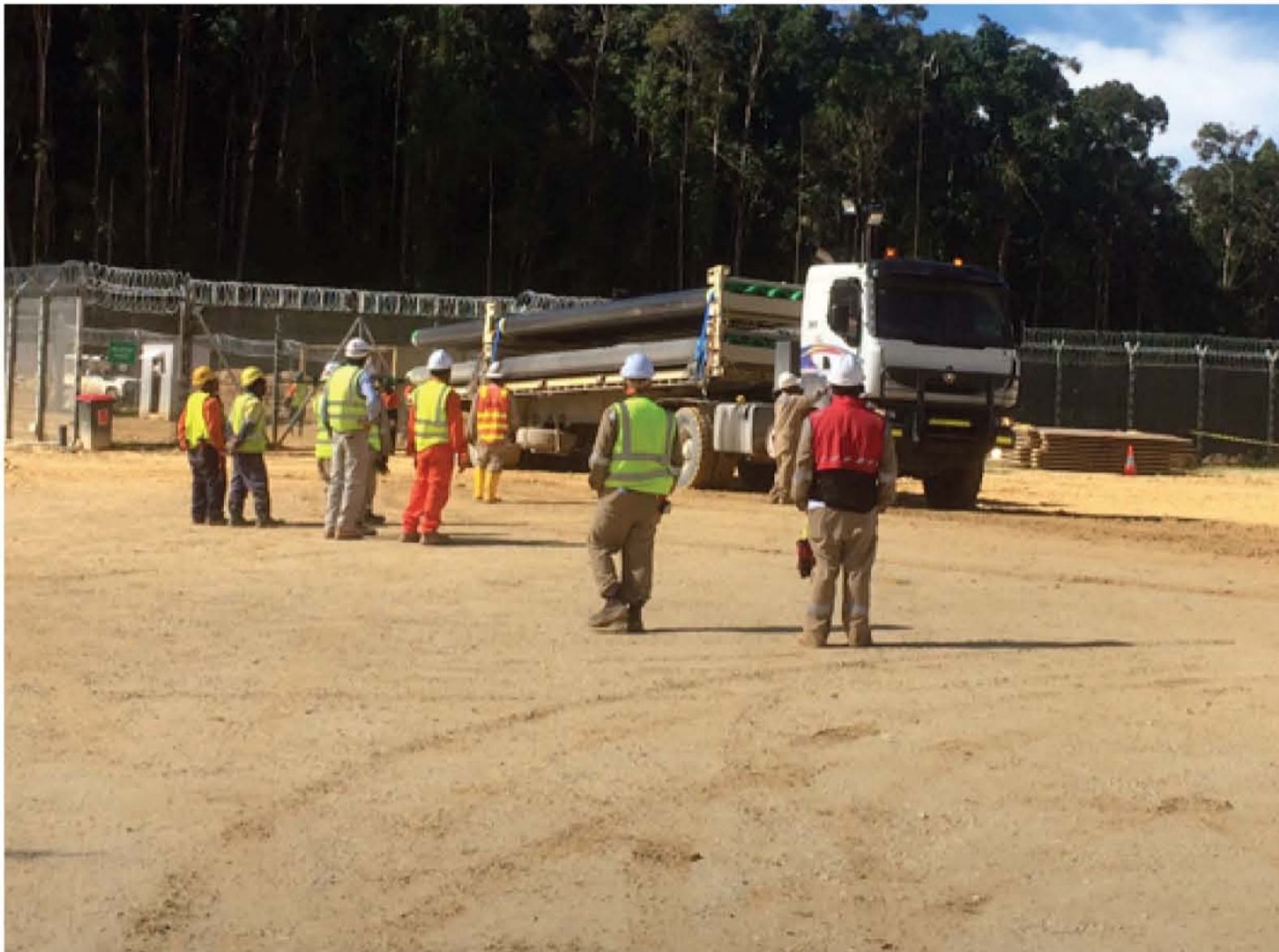
Line-pipe road transport convoy arriving at Angore Wellpad A.
