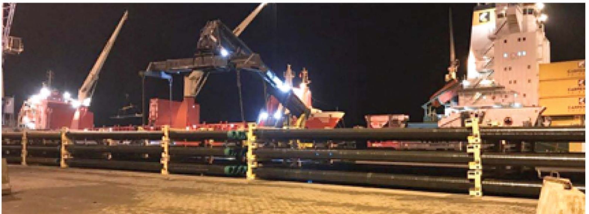
Unloading 14" line-pipe off the ship in Lae.
