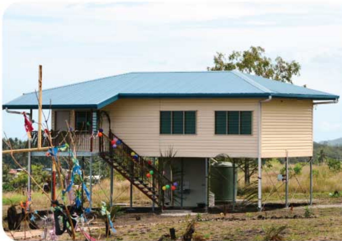
One of the newly built teachers houses funded by PNG LNG.
