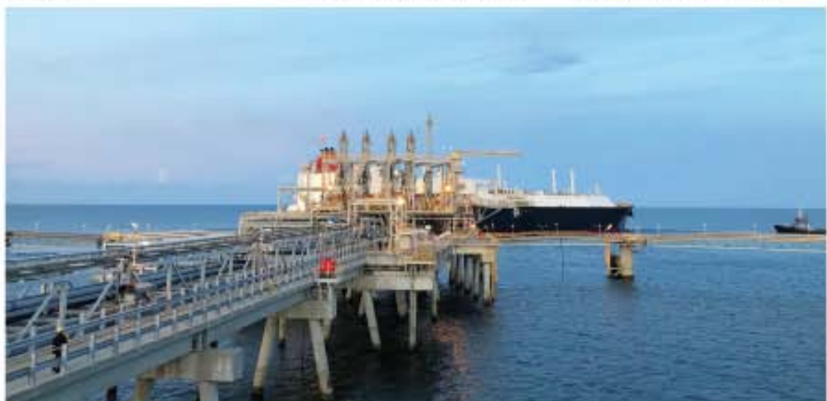
The Kumul, berthed at the marine terminal at the LNG plant, during the offload.
