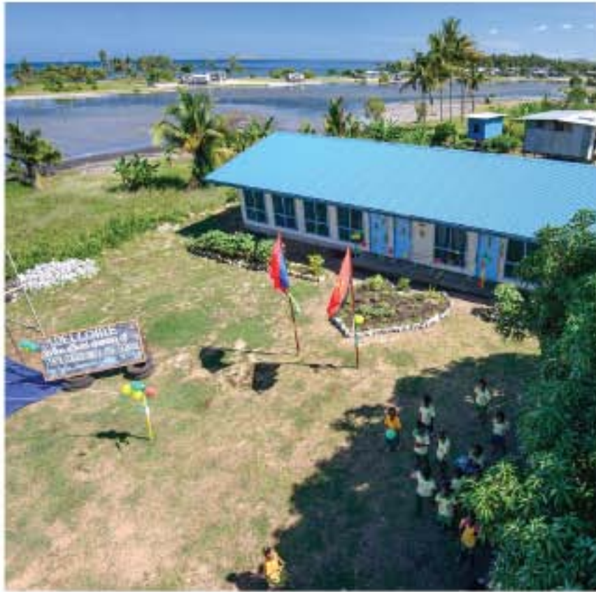
The new double classroom for Papa Community Preschool includes a teacher's office, desks, chairs and a water tank. The classroom was built by operator of the PNG LNG project, ExxonMobil PNG.
