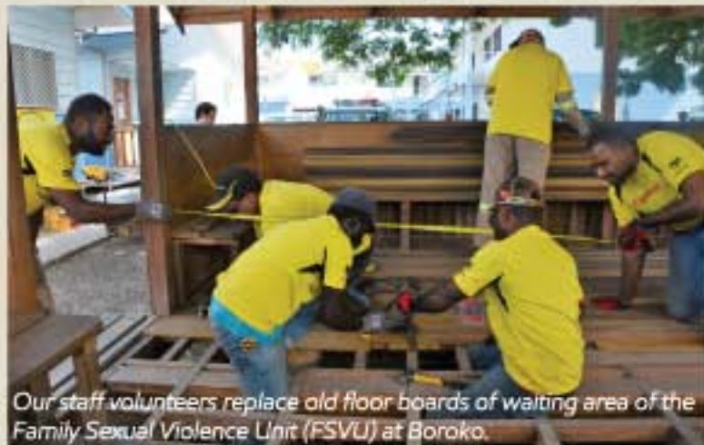
Old weathered floor boards posed a safety hazard and were removed by EMPNG staff volunteers. Rubbish that had collected over time were collected from under the building.
