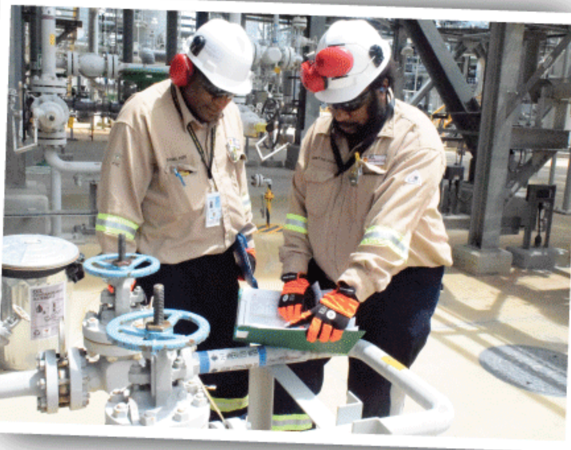
Nares technicians Daniel Pere (left) and Rodney Kuala (right) carrying out inspection at the PNG LNG plant.
