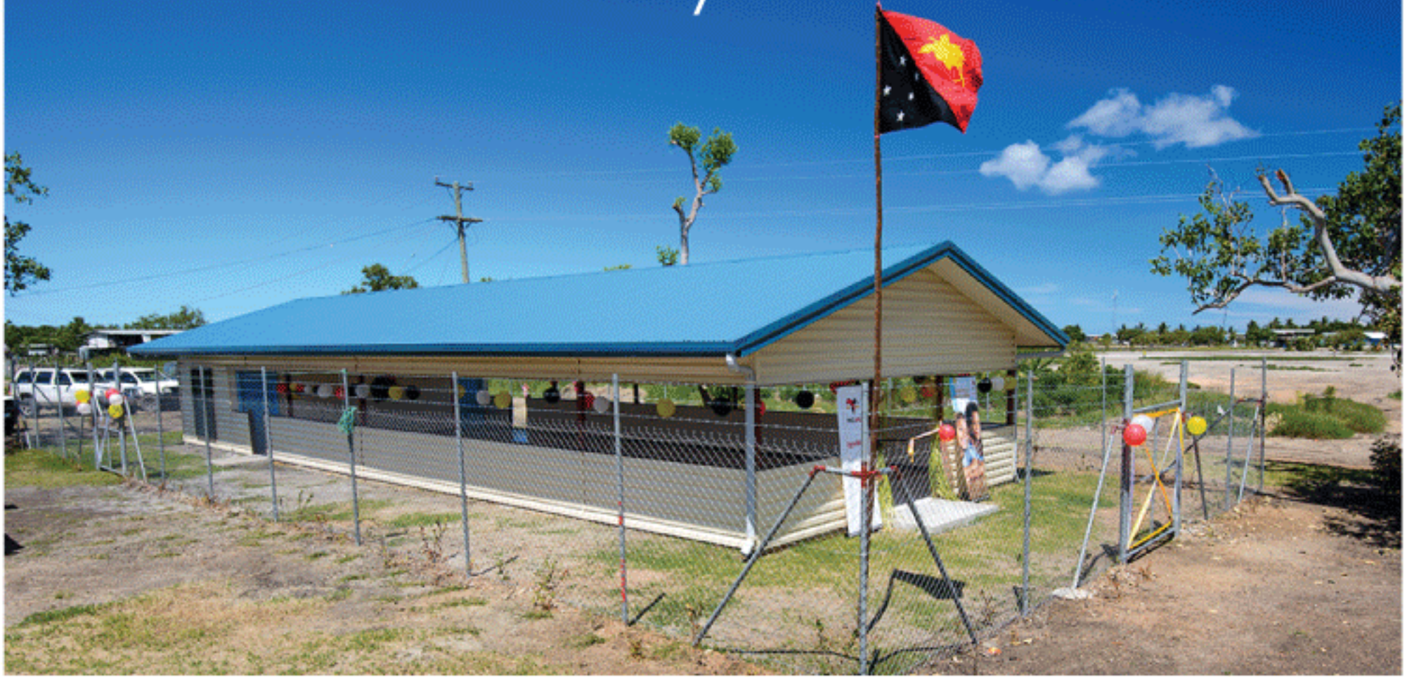
The new community hall at Lealea.
