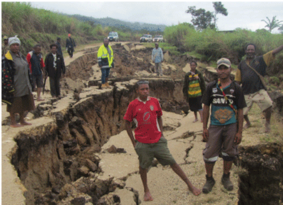
Road cracks in Anguale caused by the earthquake made it impassable for vehicles to drive through.
