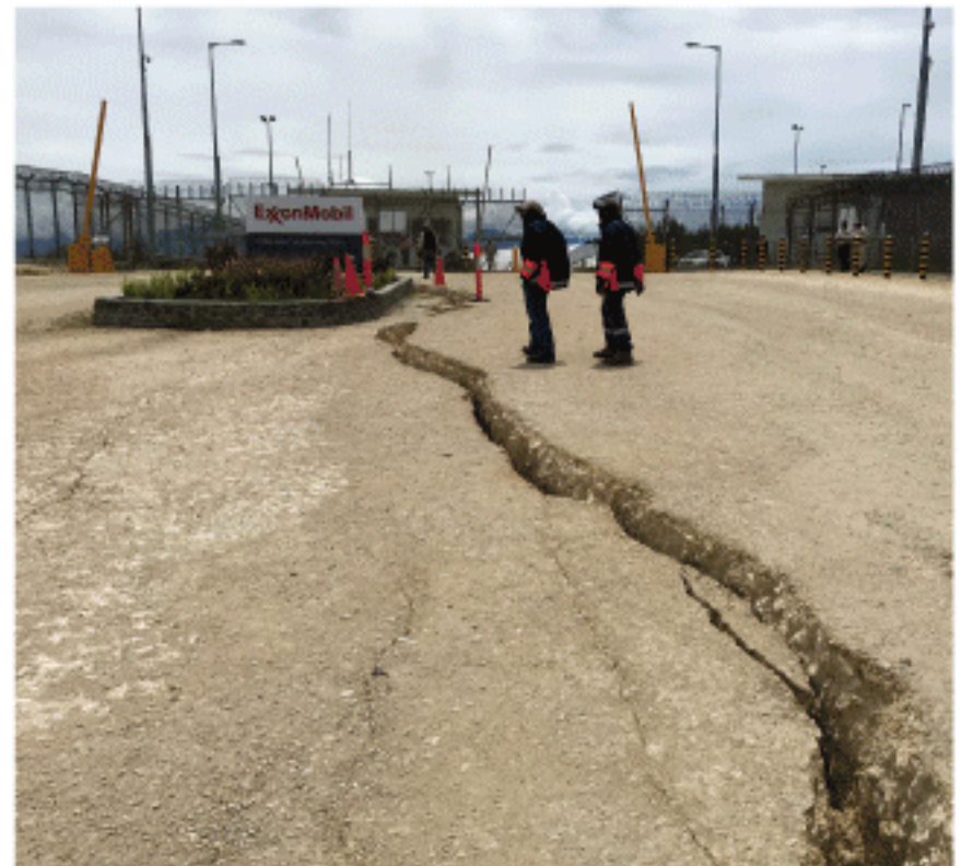
Cracks in the road at the entrance to the Hides Gas Conditioning Plant.
