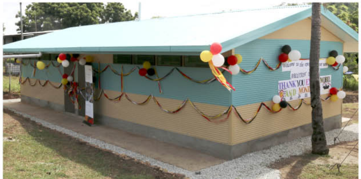
New ablution block at Boera Primary School
