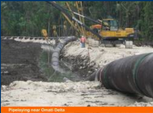
Pipelaying near Omati Delta
