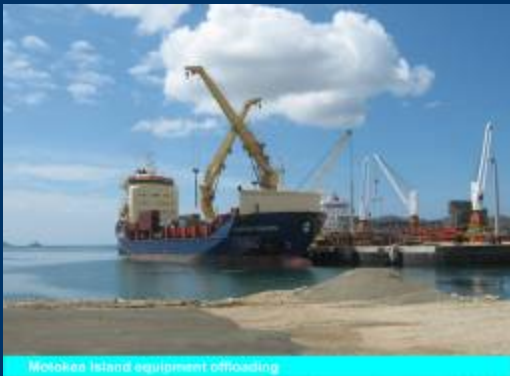
Woskes Island equipment offloading
