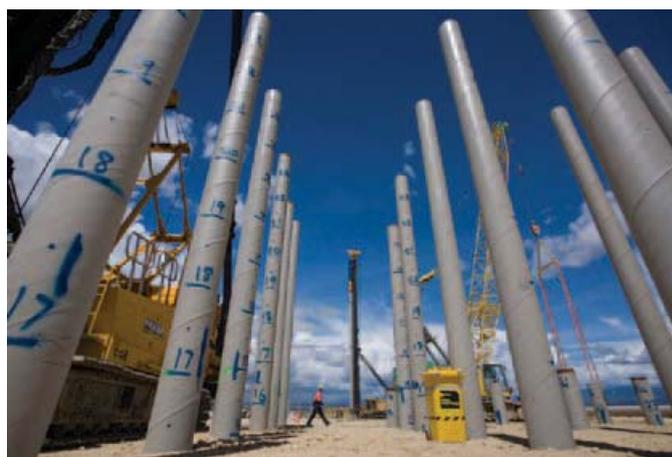
Plate 2.1 – Foundation piles for the HGCP utilities area
