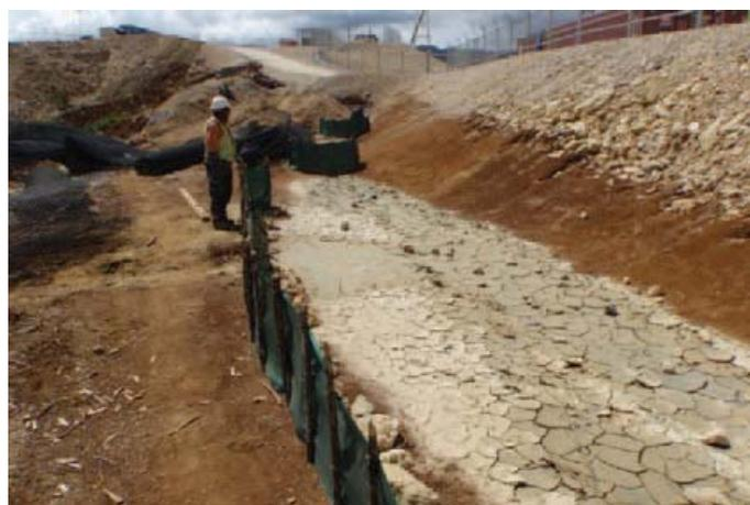
**Plate 11.1 – Erosion control structure at the HGCP site**
