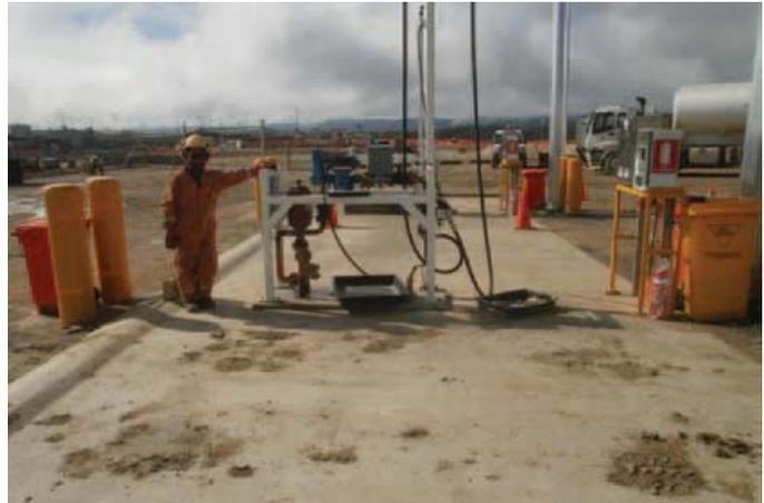
Plate 9.8 – Fuel farm showing drip trays, bunding and spill kits
