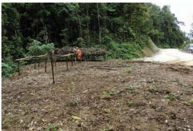
Plate 10.2 a-b – Weed control operations and weed drying platform along the Kantobo to Mubi River Road
