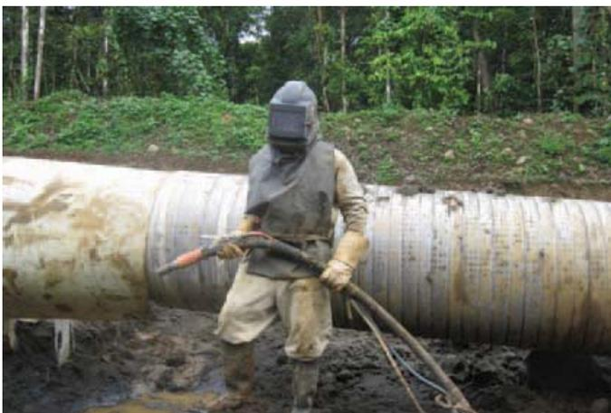
Plate 7.5 – Worker conducting abrasive blasting
