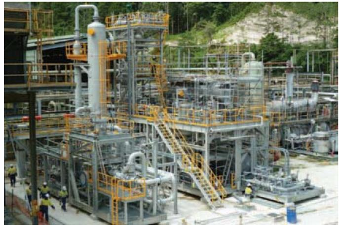
Plate 2.6 – Triethylene glycol module
