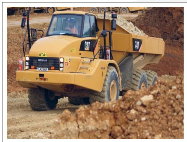
Bulk earthworks at the Hides Gas Conditioning Plant continue
